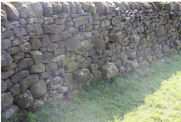
The east wall is built of gritstone. A wide gate has been cut through the wall, but the remains of the wall, original foundation are still visible. SE 00136 53563
