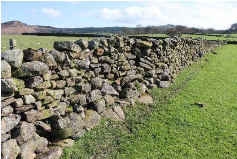
The north wall is built of gritstone including some large 'cobbles', some of which have been made smaller during wall reconstruction.
