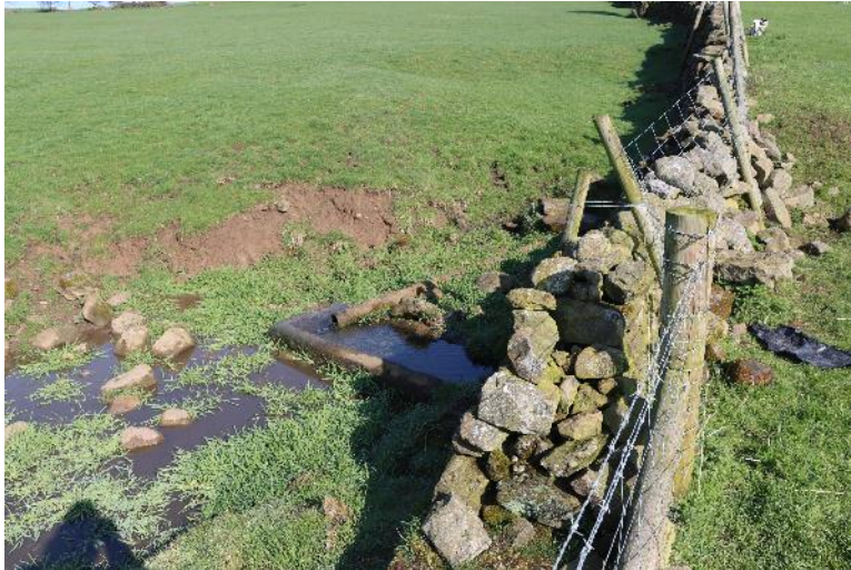
The western boundary contains a gritstone wall, with ditch to the west with a spring running down it. A stone trough collects water from the spring and a drainage pipe exits to the trough. SD 99996 53535
